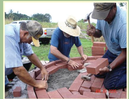
also installed. A rock and cement trough was built in the front to accommodate the coals that are dragged out of the oven before the bread is baked. The oven was left to dry for about a month and the rebar was taken out.
